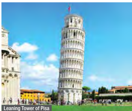
Leaning Tower of Pisa
